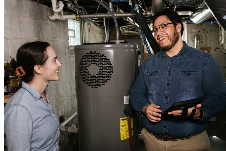
HVAC System Upgrades
