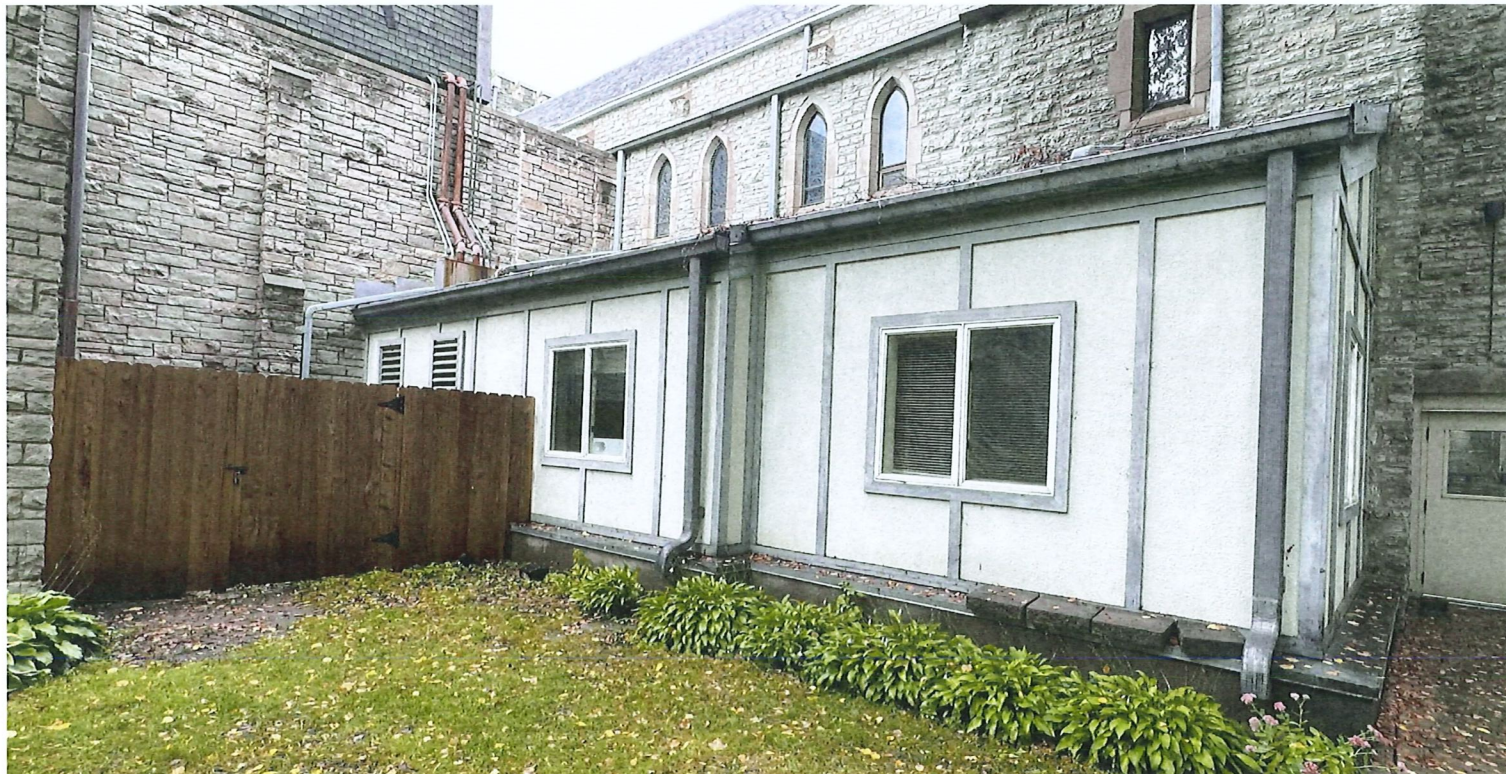
EXISTING ROOM ADJACENT TO CREEK TO BE REMOVED
