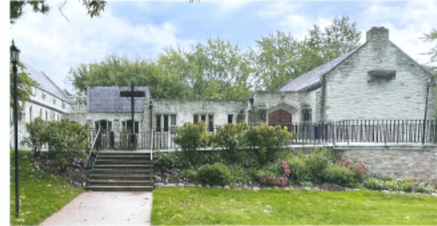
ENTRANCE WITH ACCESSIBILITY CHALLENGES & EXISTING ROOFTOP EQUIPMENT ENCLOSURE
