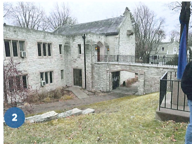
CHAPEL ENTRY RAMP ( APPROX. 1:19) MAY BE NON-COMPLIANT, AND DIFFICULT TO MANEUVER IN WINTER
