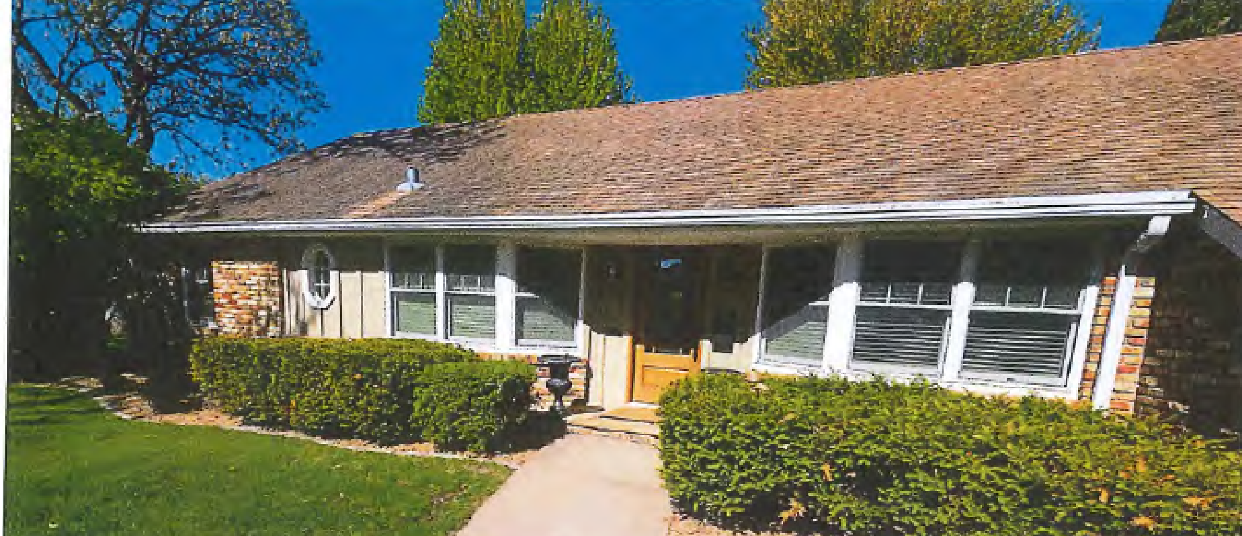
Close up photo of the existing front façade
